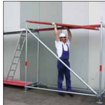
Assemble decks from lower level
