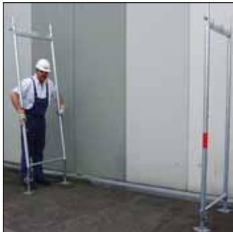
Assemble vertical frame
