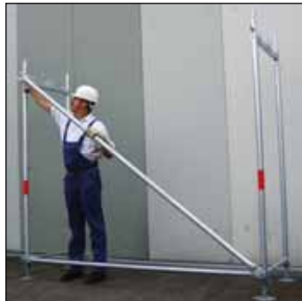
Assemble vertical brace
